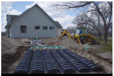
*Conventional gravity fed septic system with concrete tank and distribution box. Drainfield is a bed configuration with graveless chambers.*
